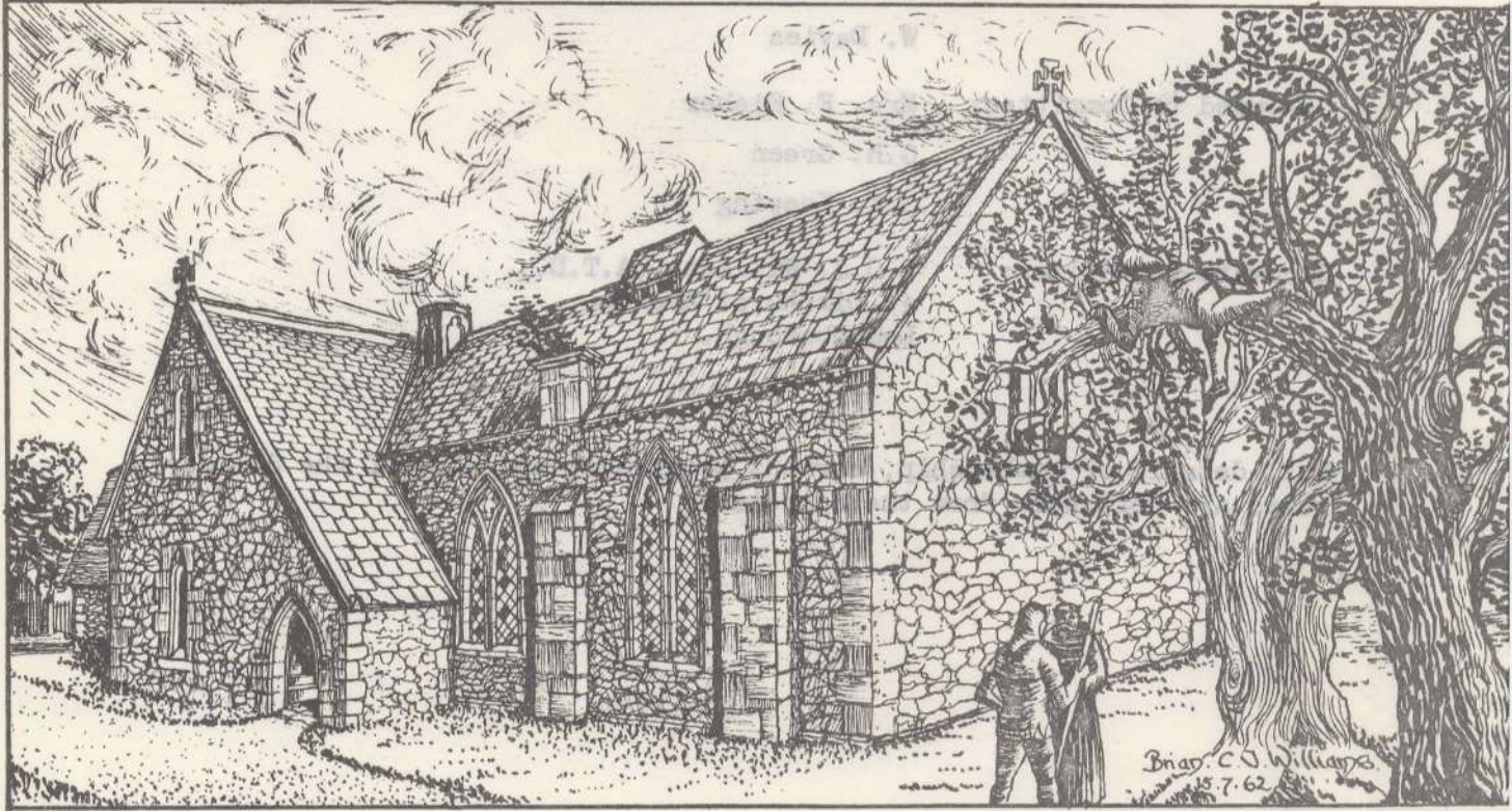
A 14th century restoration view of the Old Rectory back Loughborough (Looking East)
